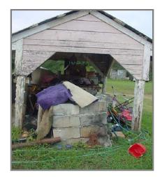
Unused water wells that are not properly abandoned leave open holes in the ground. These holes are dangerous. People (especially children), pets, and wild animals can get hurt or trapped after falling into an abandoned well. These holes serve as direct channels for contamination into Georgia's groundwater. They allow chemicals and bacteria from the surface environment to pass straight through to a drinking water source used by many people.
